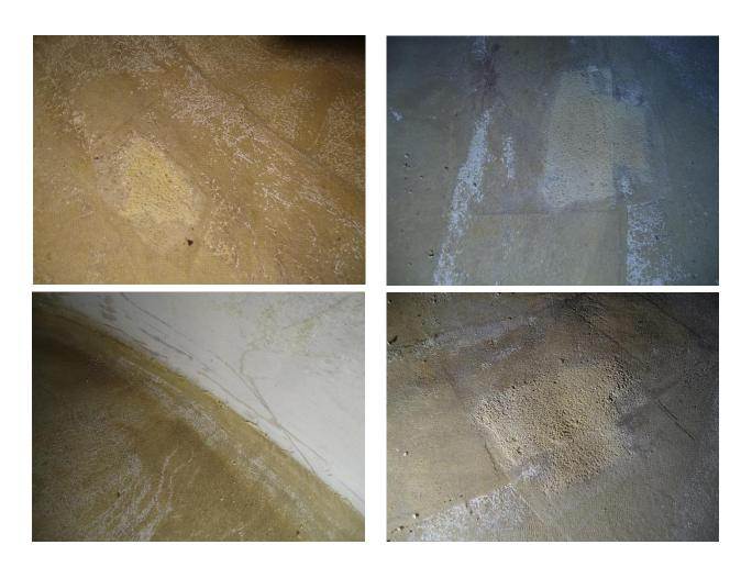
Photo Set 9: Close up view of the dryness and roughness of the tank floor
