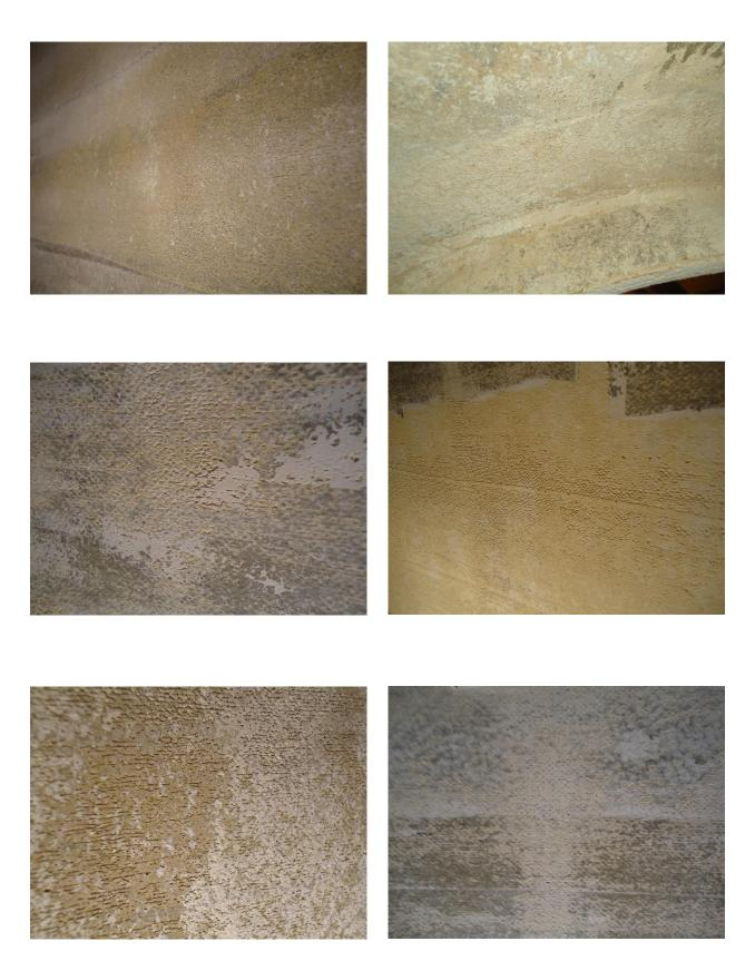
Photo Set 11: Close up view of the dryness and roughness of the tank wall
