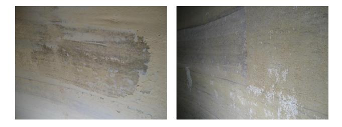
Photo Set 10: Close up view of the dryness and roughness of the tank wall
