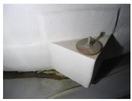
Photo Set 2: Tank hold down lugs: appear to be structurally sound
