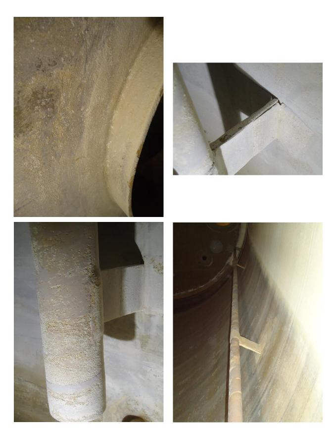
Photo Set 13: Manway stub and downpipe condition (inside)
